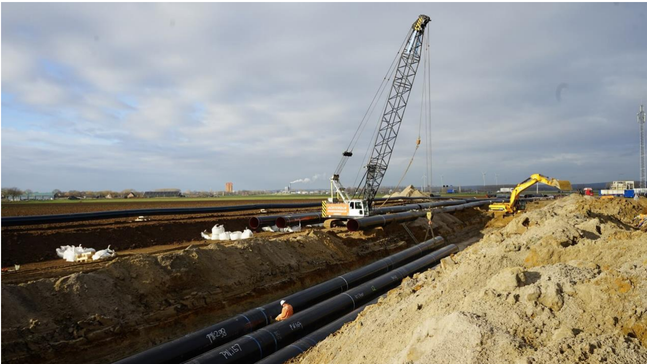
Relocation of cables and pipelines before the start of the construction works of the ViA15 highway missing link © Rijkswaterstaat
