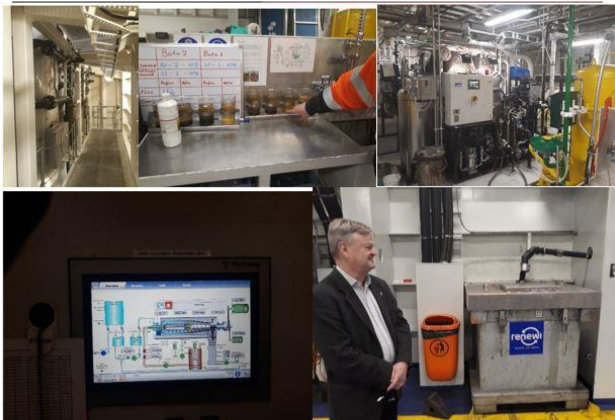
Scrubber installations on the Stena Hollandica ferry © INEA
