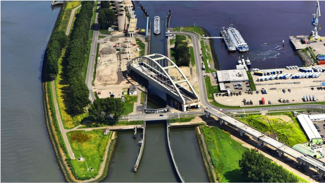
One of two new steel bridges and the continuation on the concrete substructure of the new Theemsweg rail section in the Port of Rotterdam (NL) © PoR
